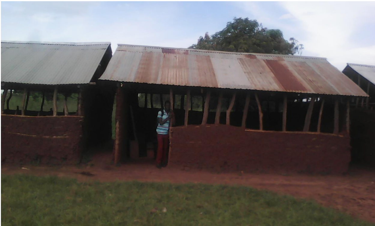
Figure 3 Mud made classroom blocks constructed for the lower section/younger pupils
