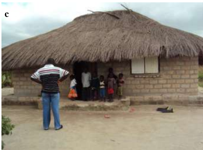
Figure 2 a. Remnants of the affected house after it was burnt by fire caused by lightning b. Police officers shows the place where they found the bodies after they were pulled out by Mr Siame c The affected house was very similar to this before being burnt by fire
