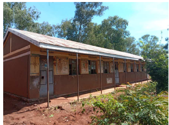
Figure 3. Veranda poles on Mongoyo Classroom Block C
