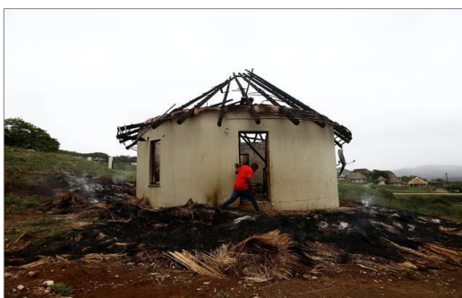
Fig. 4. Rondavel where people died, perhaps from the lightning strike but complicated by the fire caused when the thatch caught fire and fell on them.
