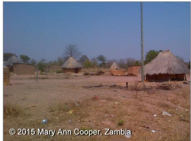
Fig 1. Typical African dwellings and work areas are mudbrick with generations-old thatch roofs or sheet metal held down by rocks. In some areas, chicken wire may be cast over the thatch to prevent monkeys and baboons from disrupting the roof. In others, car tires are on the roof because it is thought that their ‘rubber’ will protect the building from lightning.
