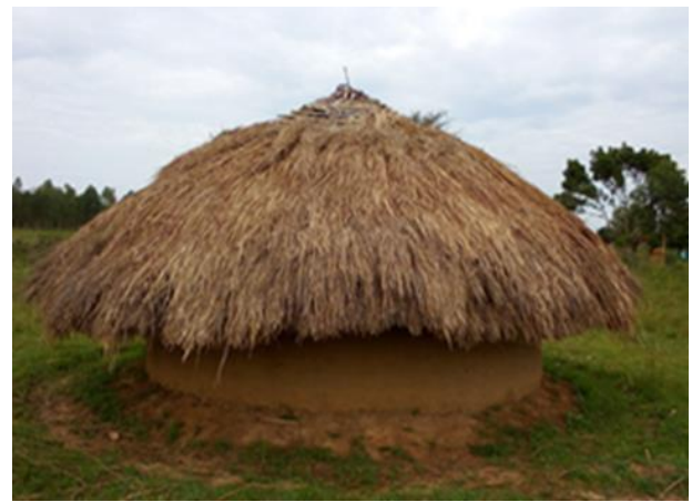
Fig. 2. Most of the children who were injured were attempting to take shelter from the drizzle by sitting on a small veranda or bench seen at the base of this unfinished hut. The top center point of the roof was not yet thatched so that rain and sunlight could penetrate to the inside.
