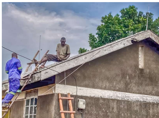
ACLENet installing a lightning protection (LP) system atop a Ugandan school building, including the vertical air terminals (lightning rods), connectors and down conductors to a properly engineered earthing ring about the structure. LP systems do not prevent lightning strikes - they provide a means for the current to flow harmlessly into the ground.
